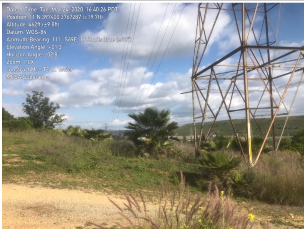
Between the towers looking East.
