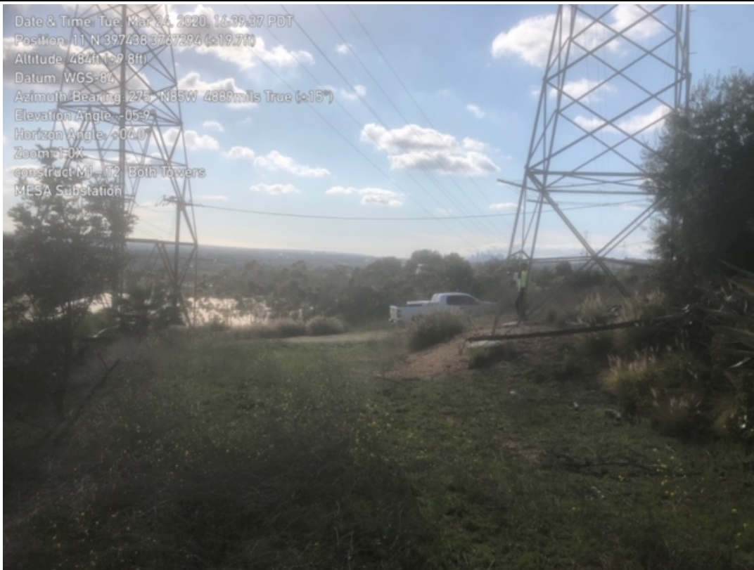
Between the towers looking West.
